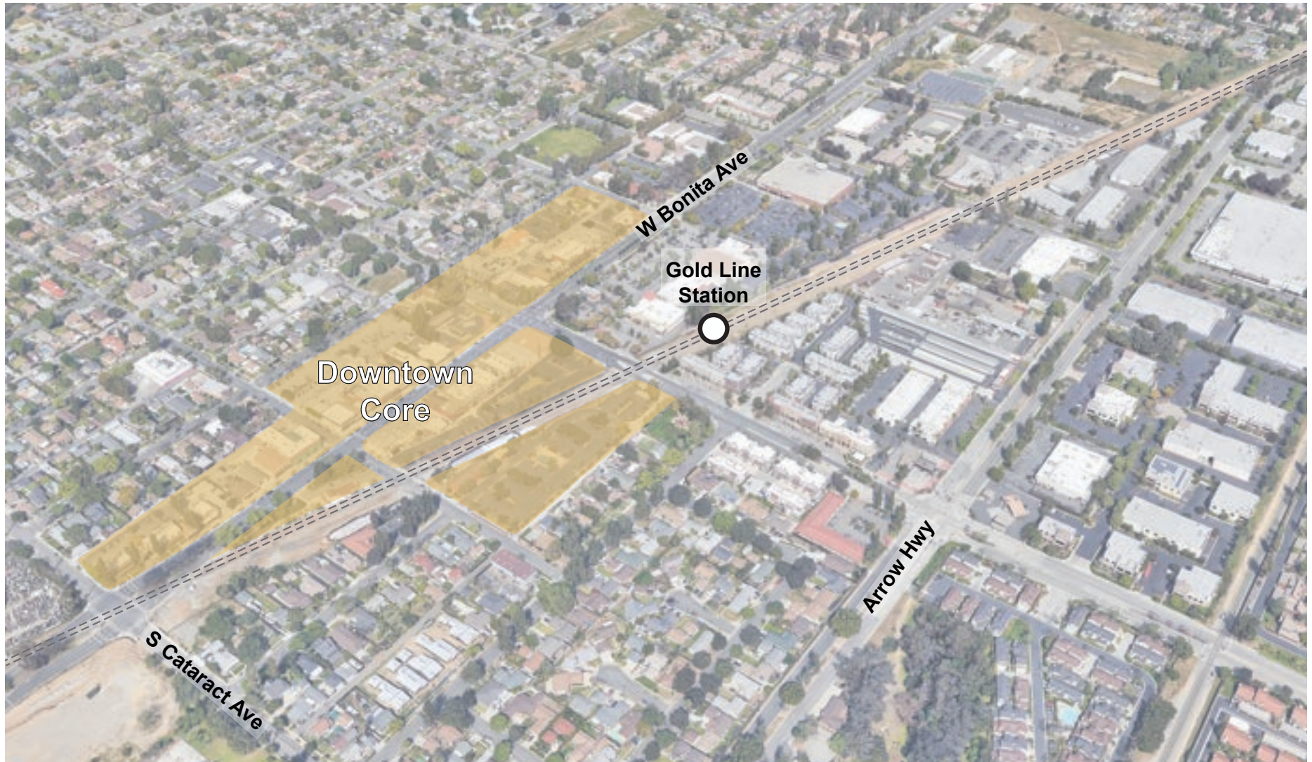
Figure 1.2-2: Aerial Photo of Downtown Core
